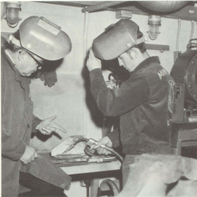
Mr. Bruhn instructs Paul Kelzer on proper use of new mig welding machine.
